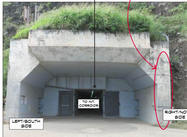
4 EXTERIOR FACADE OF BUNKER LOCATION PHOTO
