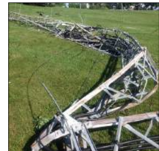
REF - FALLEN ANTENNA TRUSS
