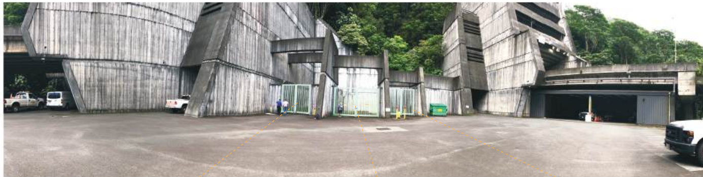
H3 LOWER TUNNEL LOCATION
